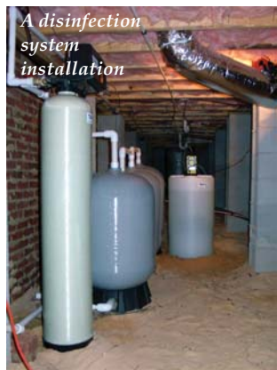
Here, Bradley used open-air oxidation and filtration for problematic waters
